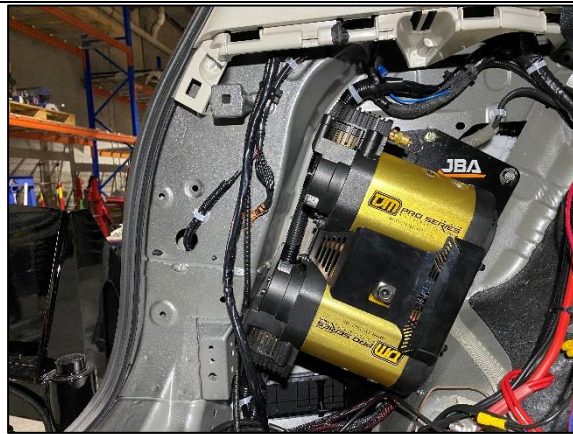
STEP 5.9 NEATLY CABLE TIE AND LOOSE LOOMS AND AIR LINES. TEST ALL AIR CONNECTIONS FOR AIR LEAKS AND CYCLE COMPRESSOR CHECKING ELECTRICAL FUNCTIONALITY.
