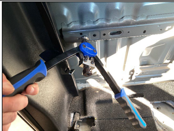
STEP 1.15 INSTALL 2 X M6 CAPTIVE RIV NUTS SUPPLIES IN THE TO DRILLED LOCATIONS.
