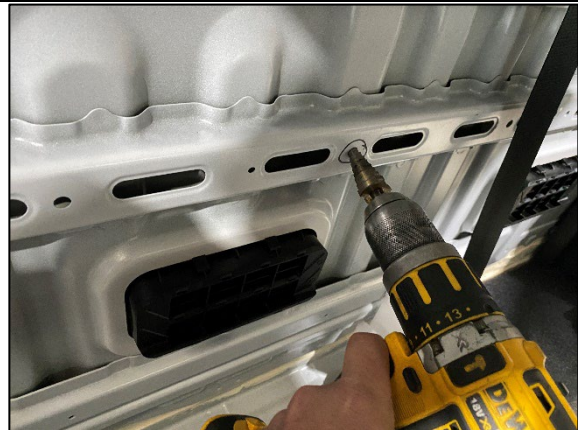
STEP 1.14 DRILL OUT THE MARKED 2 X HOLES TO 10MM.
