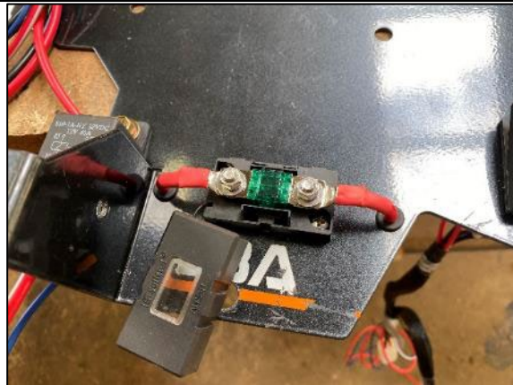
STEP 2.7 CRIMP THE CABLE LUGS ON TO THE WIRE ENDS AND HEAT THE HEAT SHRINK AS SHOWN.
